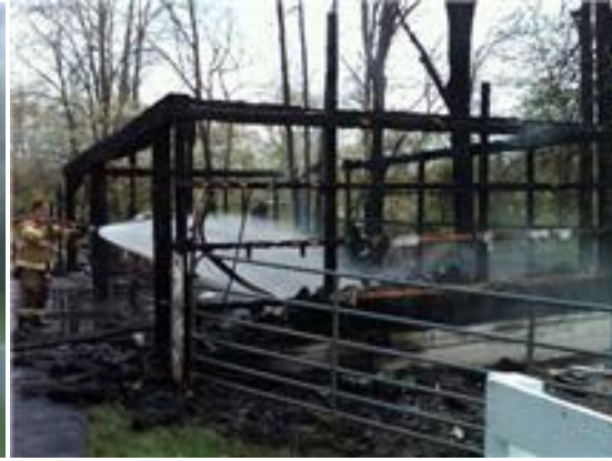
Well involved garage fire. Vehicles saved, structure was a total loss
